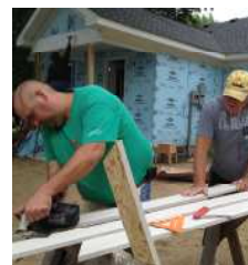
Bob Uhrick & Maurice Nickels cut trim boards
